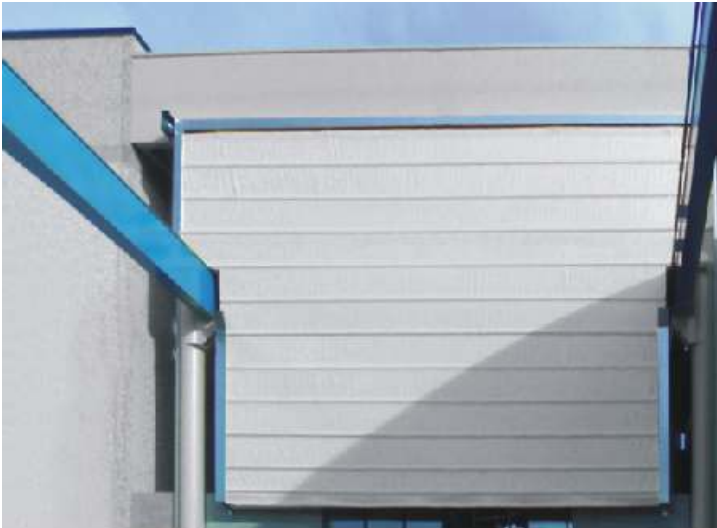
Fixed Crane Accesses
