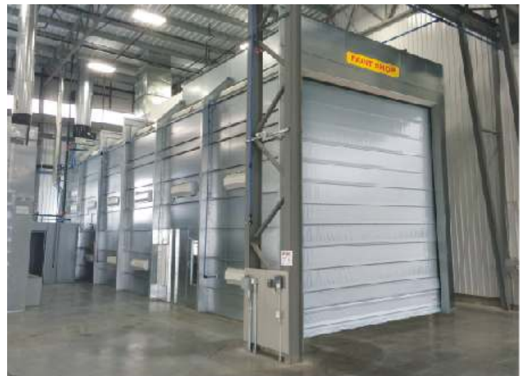
Sand-blasting and Paint Hangars
